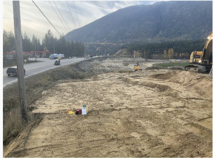
Photo 6: Site EeQt-84 Excavation across from Co-Op
