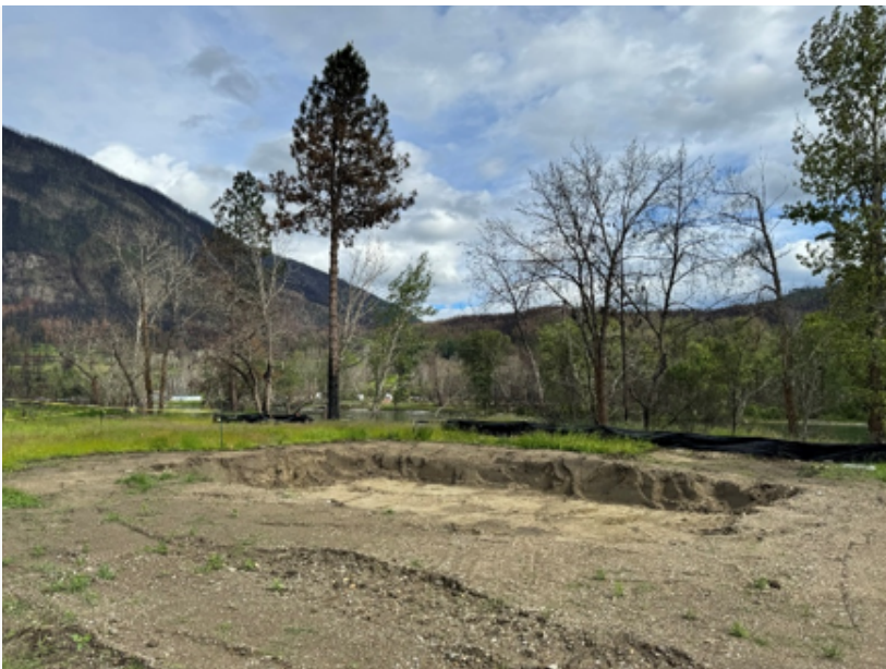
Figure 4 Excavating contaminated soils
