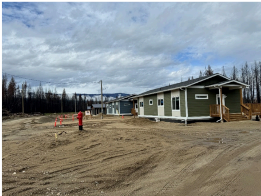
Figure 1 LSL Road East looking eastward
