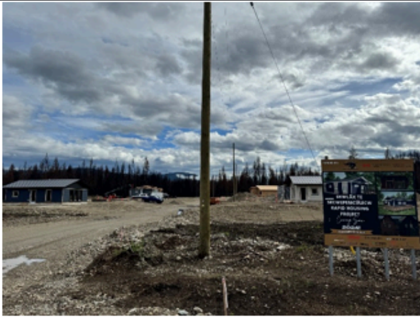
Figure 3 North subdivision under construction
