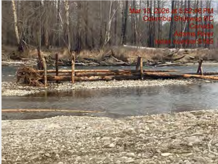
Photo 3. A Post Assisted Log Structure (PALS) installed in the Lower Adams River to increase salmon and trout spawning habitat.
