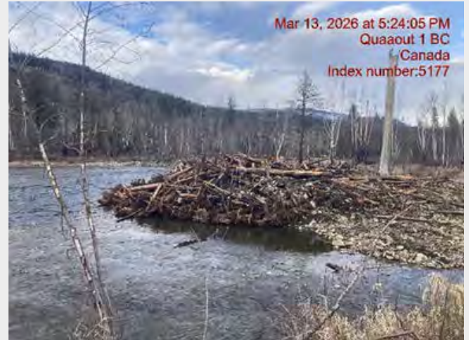
Photo 1. One of three woody structures placed at the upstream end two side channels that was widened at its' upstream end to draw more flow.
